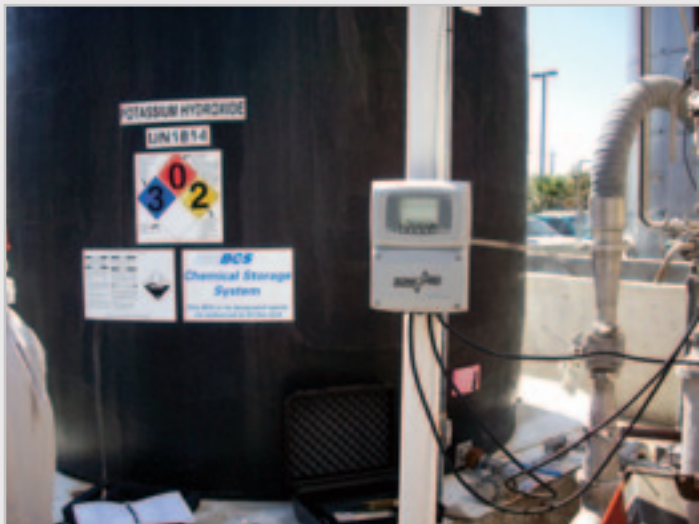
Sonic-Pro's ability to measure corrosive fluids from outside the pipe made it the perfect choice for this food processing plant's potassium hydroxide application.
