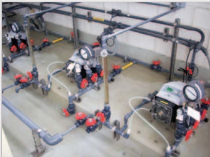
Flex-Pro cannot vapor lock in this chloramine application.
