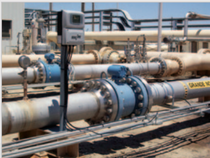
Sonic-Pro quickly installed on this 10" 316 stainless steel water flood injection line resulting in zero down time on this 50,000 barrel per day oil production application.
