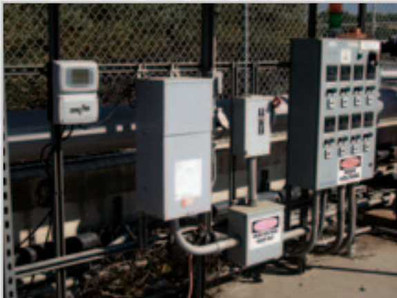
Sonic-Pro clamp-on ultrasonic flowmeter, solves the problem of fluid measurement where there is sludge build-up, in this groundwater remediation application.
