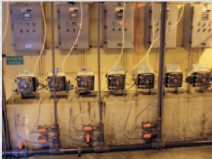
Chlorine dosing at this municipality is much more precise, accurate, and consistent using a peristaltic pump rather than a pulsating pump. The operator was impressed at how easily the peristaltic pump hooked into their SCADA system.
